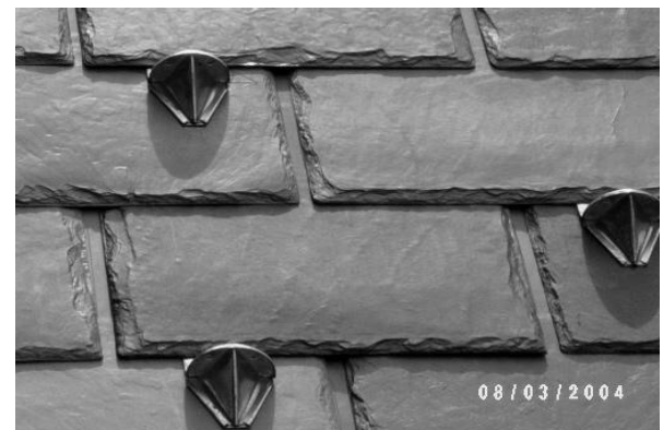
The new snow guards on the Grace roof.
